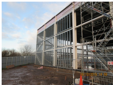
Photograph 11 Following completion of main structural steelwork the steel erector has now commenced the erection of the external steel partition frame. First works on the sports hall.
