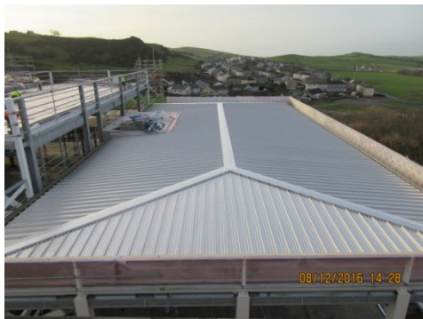
Photograph 1 Sports Hall Roof Complete
