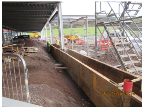
Photograph 9 Perimeter formwork shutter being installed for the ground floor slab between grid point E and J(1)
