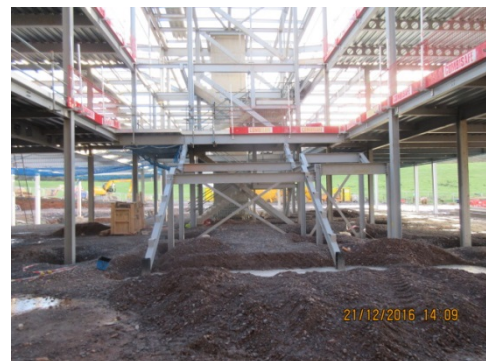
Photograph 12 First view of the Atrium staircase from ground level
