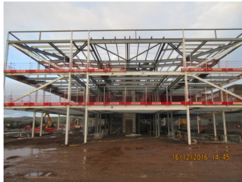
Photograph 7 – The South gable end of the new school building. This marks the completion of the structural steelwork.
