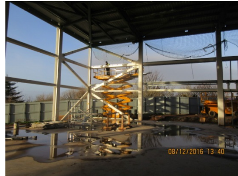
Photograph 6 Steel erector carrying out paint remediation. When the steel is chained for lifting into position the paint protection is "rubbed" off. The paint is reapplied when the steel is in situ.
